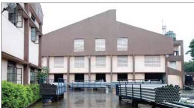
DADRA - SILVASSA PIPES & WATER TANKS
