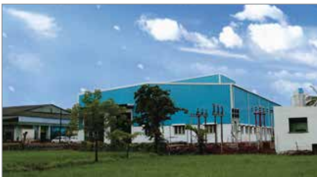
CHENNAI - TAMIL NADU PIPES
