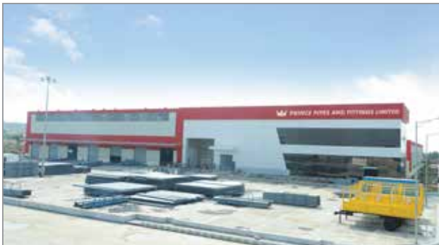
JOBNER - RAJASTHAN PIPES & WATER TANKS
