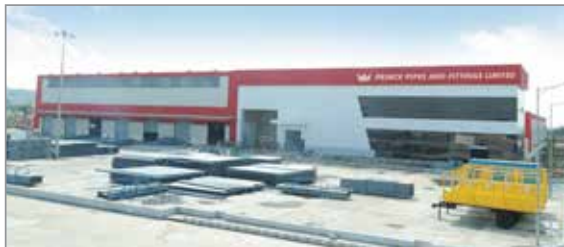
JOBNER - RAJASTHAN PIPES & WATER TANKS
