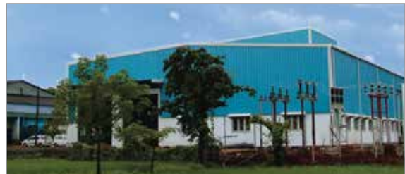
KOLHAPUR - MAHARASHTRA PIPES
