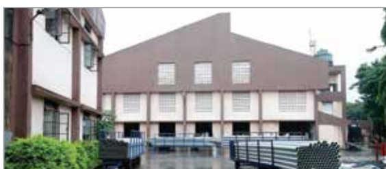
DADRA - SILVASSA PIPES & WATER TANKS
