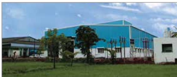
CHENNAI - TAMIL NADU PIPES
