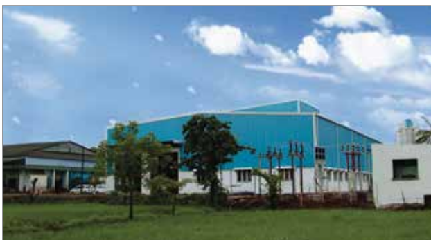
CHENNAI - TAMIL NADU PIPES
