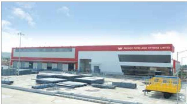
JOBNER - RAJASTHAN PIPES & WATER TANKS
