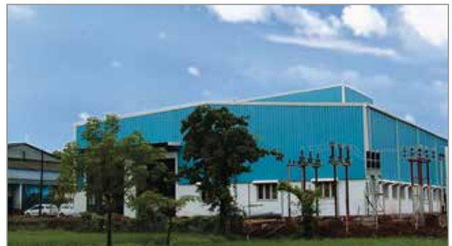
KOLHAPUR - MAHARASHTRA PIPES
