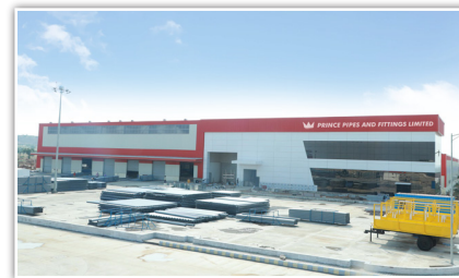
Jobner - Rajasthan (Pipes & Water Tanks)
