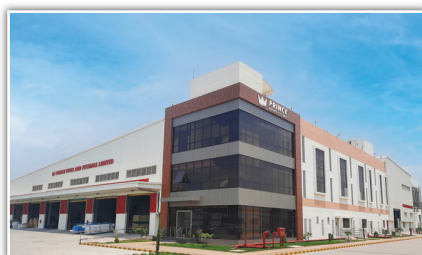
Sangareddy - Telangana (Pipes, Fittings & Water Tank)
